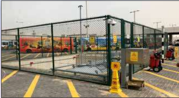
Fuel Depot Station at Dubai Parks
